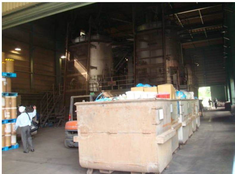
Figure 7: Mechanism for the delivery and return of the chains and dumpsters at the Marutoku facility
