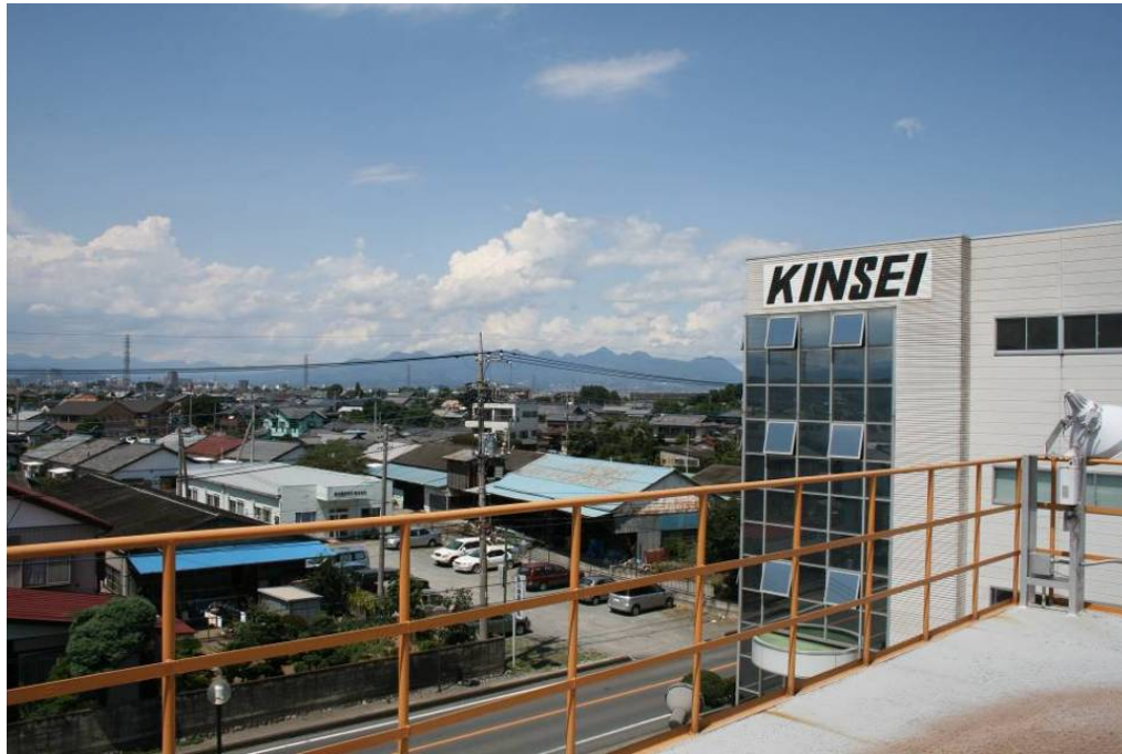
Figure 17: Kinsei Gasification Facility in Japan in close proximity to a residential area
