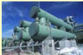
Heat / Hot Water
