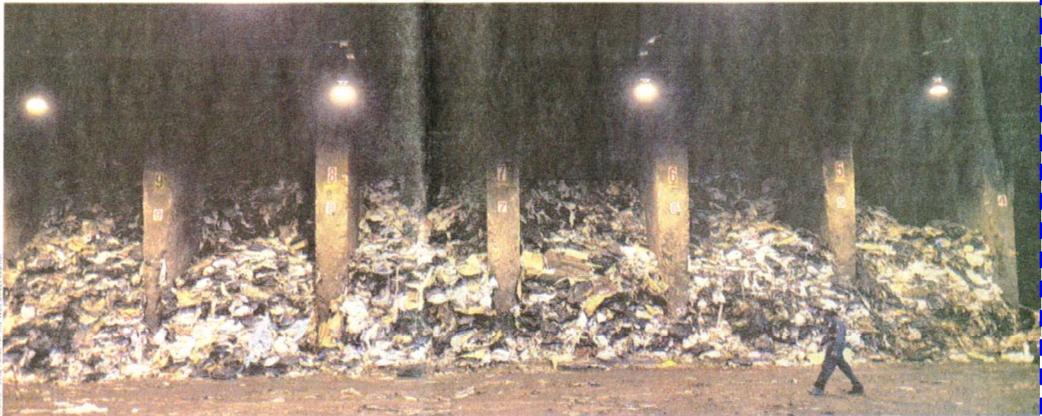
Garbage is fed into furnaces after being dropped at a loading bay at a Covanta plant in Westbury, N.Y. New incinerators are being considered in Maryland, California and Florida.
